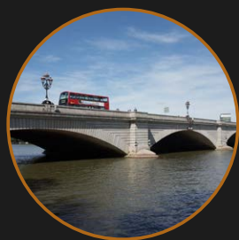
Putney Bridge 0.3 miles
